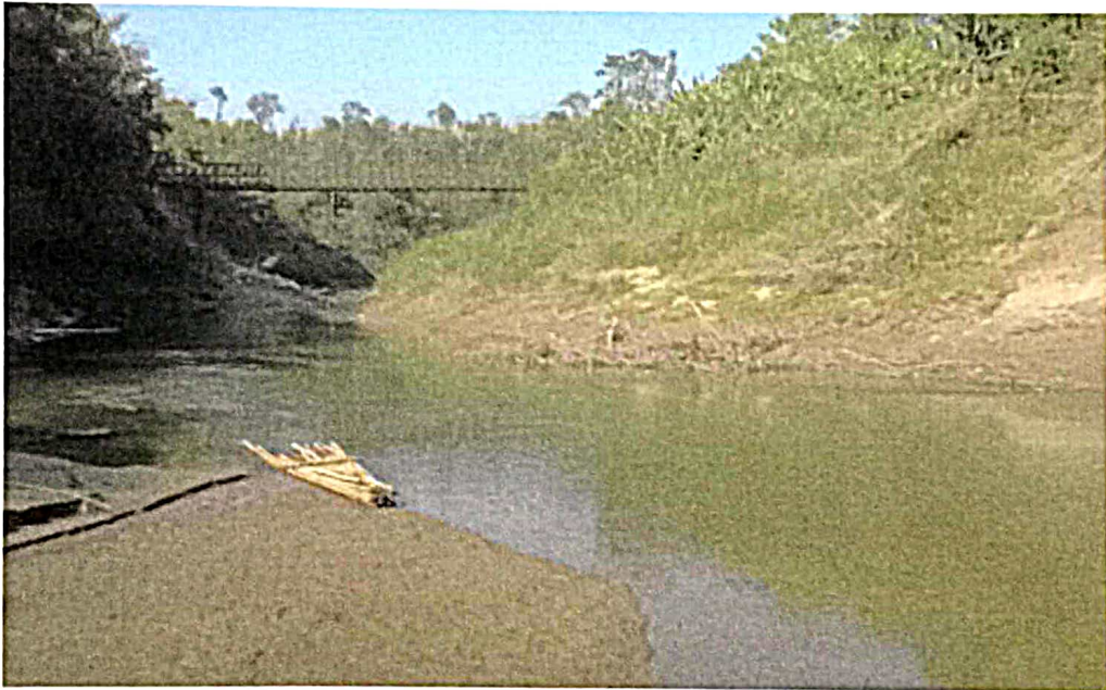
Photo plate 4.3: Site 3: Power house outlet (downstream of dam).
